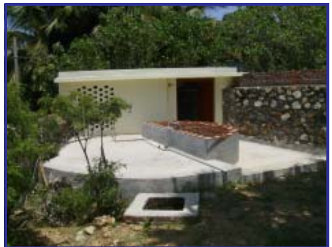
(above) Our new cement cover over our water well. It added safety to this area. Located in the building behind the water well is our 15 KV generator which "kicks-in" for unreliable local electric service.
