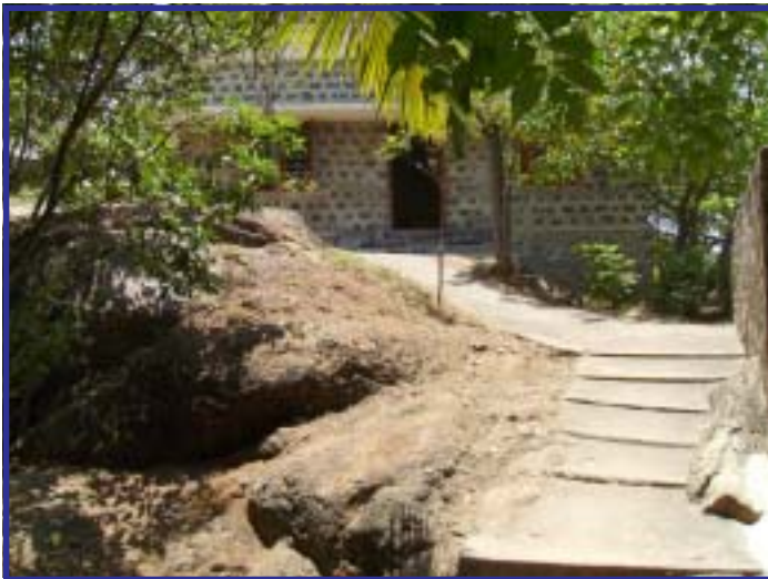
(above) Newly constructed cement walkway which leads to our Chapel. This added safety and beauty to our campus. God has blessed us with a beautiful campus too!
